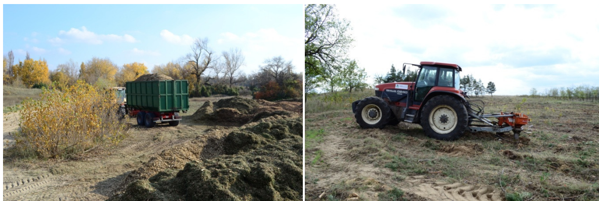
Annex 5.1.6.-3,4.: Photo on transportation of wood chips and trunk cutting
