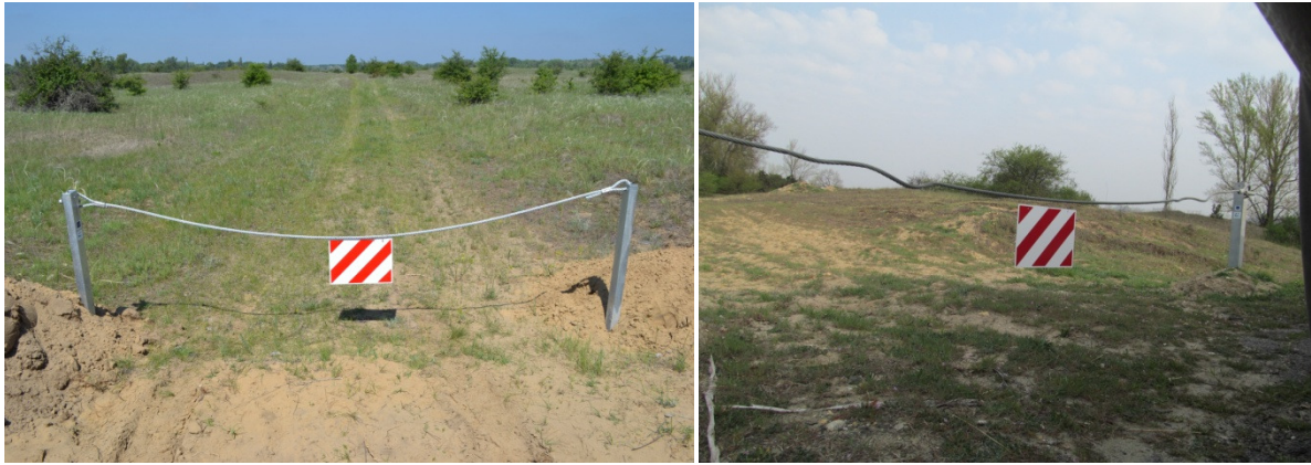
Annex 5.1.11.-1.: Photos on crossing gates
